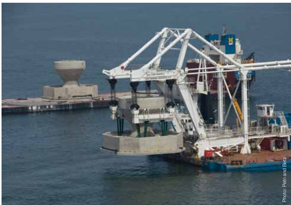
Red Sand 2 gravity base foundation - lifting operation
